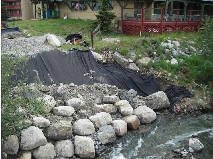
*Figure 4.5. Filter fabric installation example*
